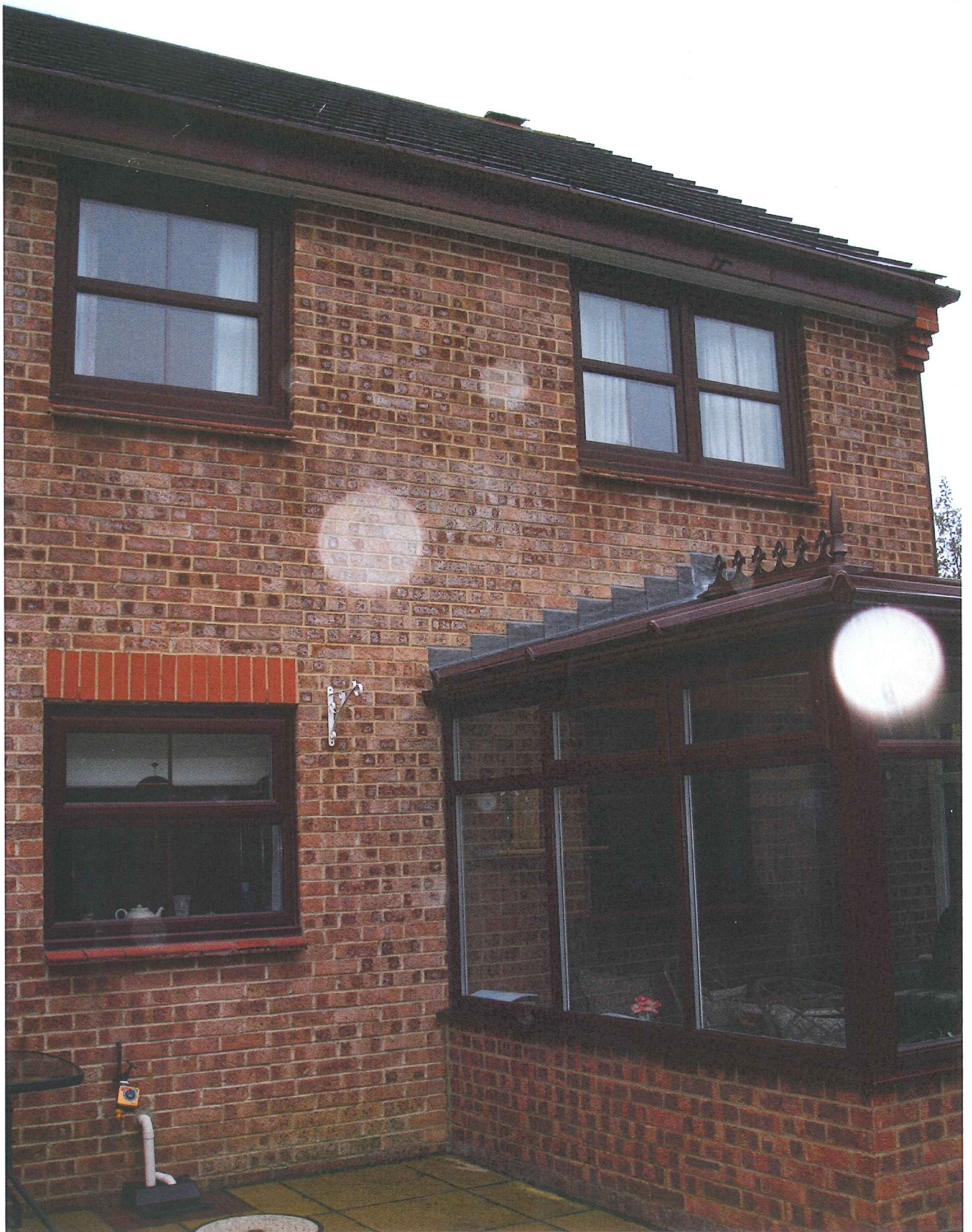
Rear of 8 New Rectory Lane
